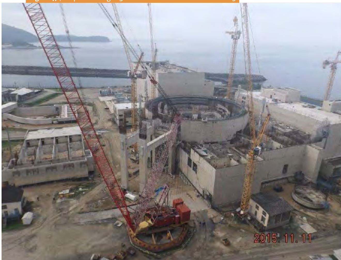
Figure 47 | Suspended Angra-3 Construction Site in November 2015
