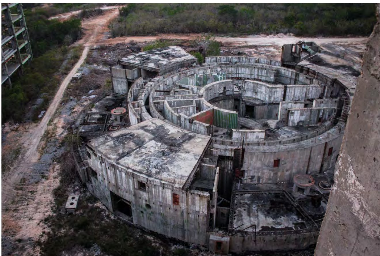
Juragua site in Cuba, where building of two Russian-designed 413 MWe reactors started in 1983 and was abandoned in 1992. Photography by © Darmon Richter, August 2014, see http://www.thebohemianblog.com/2014/08/cuba-abandoned-unfinished-soviet-nuclear-power-station.html .
